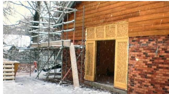
The old timber church hall was demolished in 2010 and construction of the new village hall began
